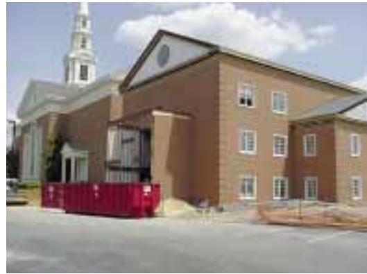
Figure 8: The Completed Addition with Successful Color Match
