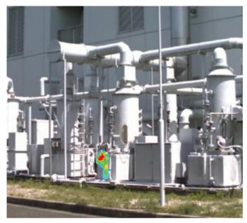
Gas monitoring solution makes gas leaks visible
