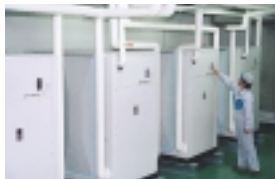
An Eco-Ice unit (ice-based heat storage heating/air conditioning system) at Itami Plant
