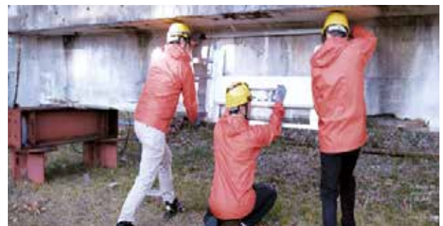
Non-destructive inspection to visualize fractures in steel materials inside a bridge
