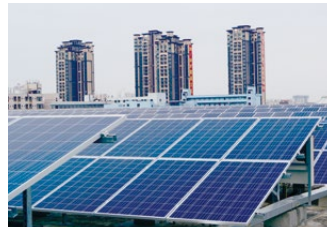
Solar power panels installed on the roof
